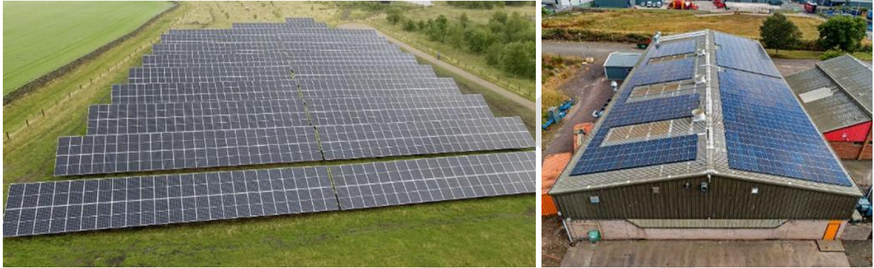
Figure 7: 500kW ground-mounted (left) 2 and 144 kW roof-mounted (right) 3
